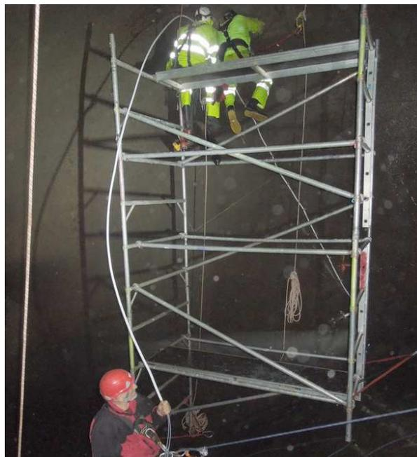
*Fig. 3. Installation of cables protection pipe in a sloping rectangular penstock (EDF Salignac HPP)*
