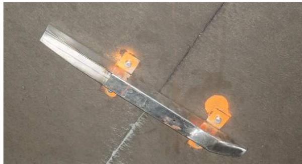
*Fig. 2. Pressure probe holder on concrete wall prepared for probe installation*
